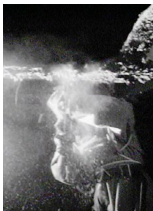
Figure 7.1 Uncontrolled dry stripping
