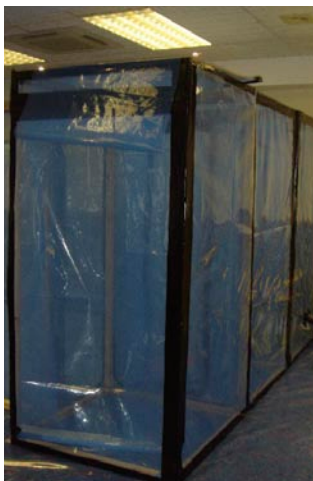
Figure 6.12 Flap arrangements for airlocks
