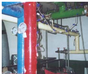
Figure 7.9 Good practice: Wet injection on pipework
