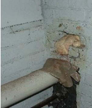
Figure 6.4 An enclosure sealed with expanding foam
