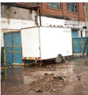
Figure 6.6 DCU attached directly to an enclosure
