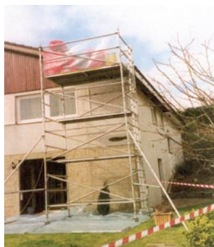
Figure 6.2 Work without an enclosure
