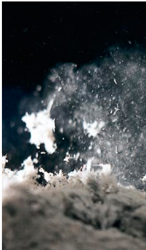
Figure 1.1 Asbestos fibres being released from lagging
