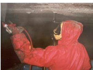
Figure 1.6 Controlled removal of asbestos
