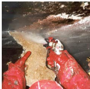
Figure 7.15 Spraying thin coating
