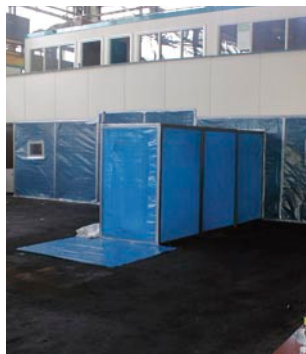
Figure 6.1 Enclosure with three-stage airlock
