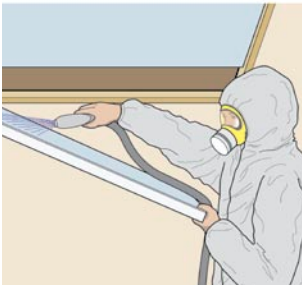
Figure 7.13 Spraying AIB
