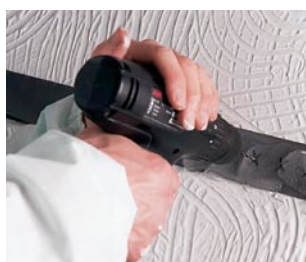
Figure 7.7 Textured coating being drilled through paste
