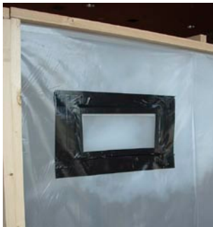
Figure 6.17 An enclosure being smoke tested
